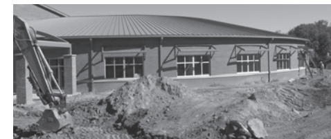
Construction is well under way at Moore Magnet.
